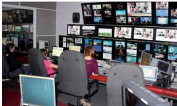
Studio control: Cabling started early March 2008 along with the installation of racks, air-conditioning and furniture
